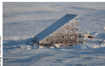
The Resolute incoherent scatter radar, located in Canada, used to measure the ionosphere.
